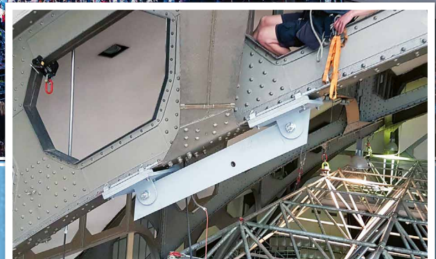
Bespoke bracketry system being installed
